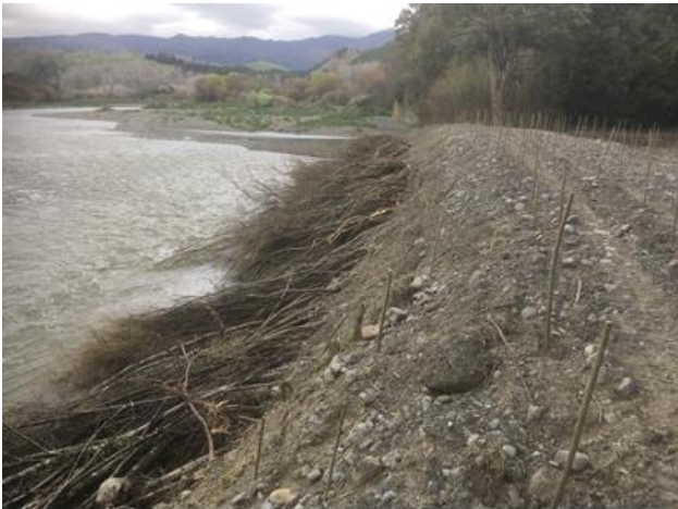
Photo 3: New flood protection wall upstream of Kahikatea campground.
